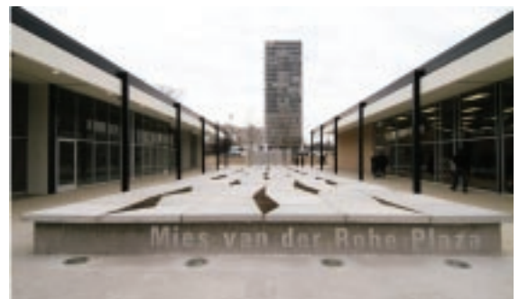
A view of the entire Mies van der Rohe Plaza looking north. In the spring, the plaza will be planted with greenery and flowers. In the background are the Lafayette Park Towers, also designed by van der Rohe.
